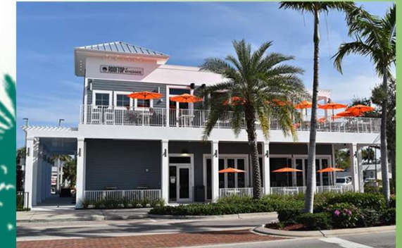
Rooftop at Riverside
