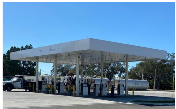
Breeze Diesel Fueling Station Source: Benesch
