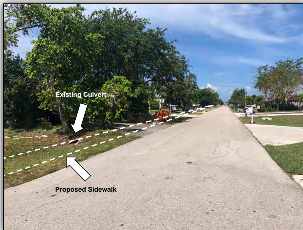
Figure 6-1: 106 th Avenue North
