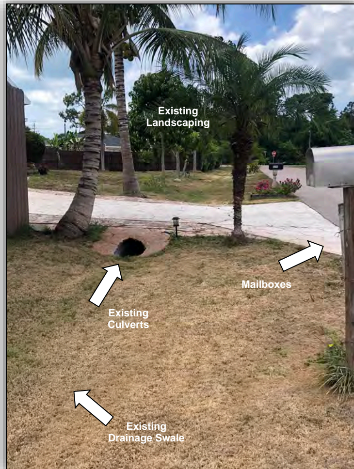
Figure 2-1: Existing Typical Roadside Ditch (Looking West)
