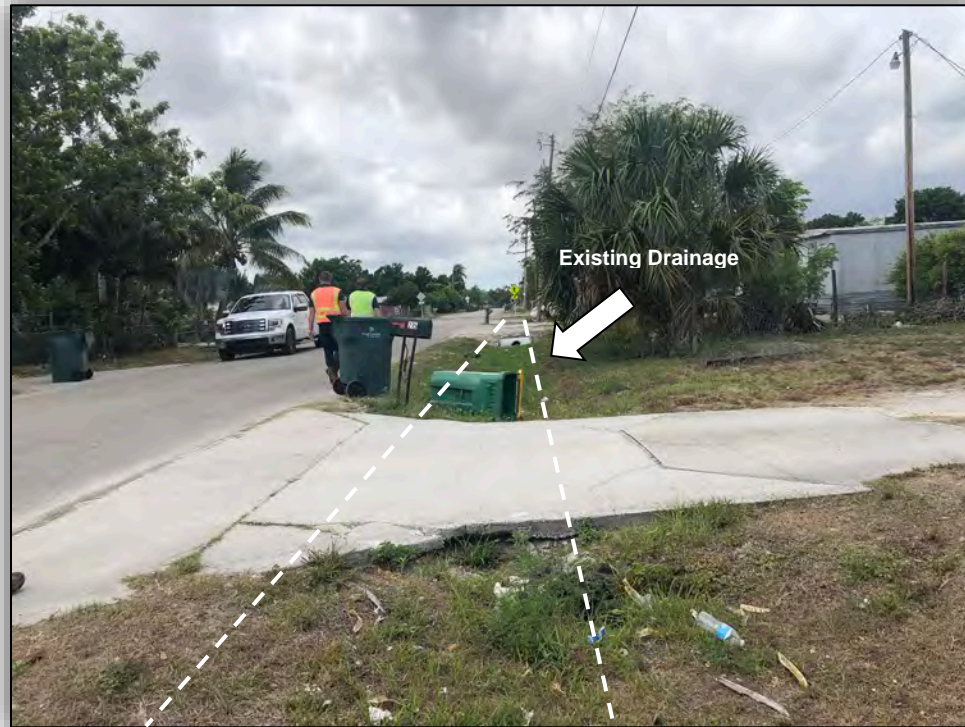
Figure 10-4: South 2 nd Street Drainage
