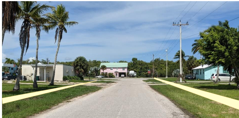
CAMELLIA STREET 75' ROW, 20' 2-LANE ROADWAY, SWALES ON SIDES
