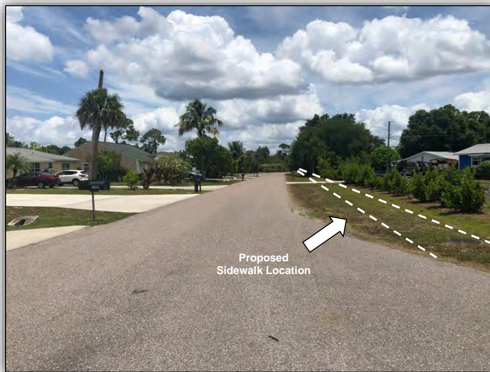
Figure 2-2: Confederate Drive Looking East Towards McCarty Street
