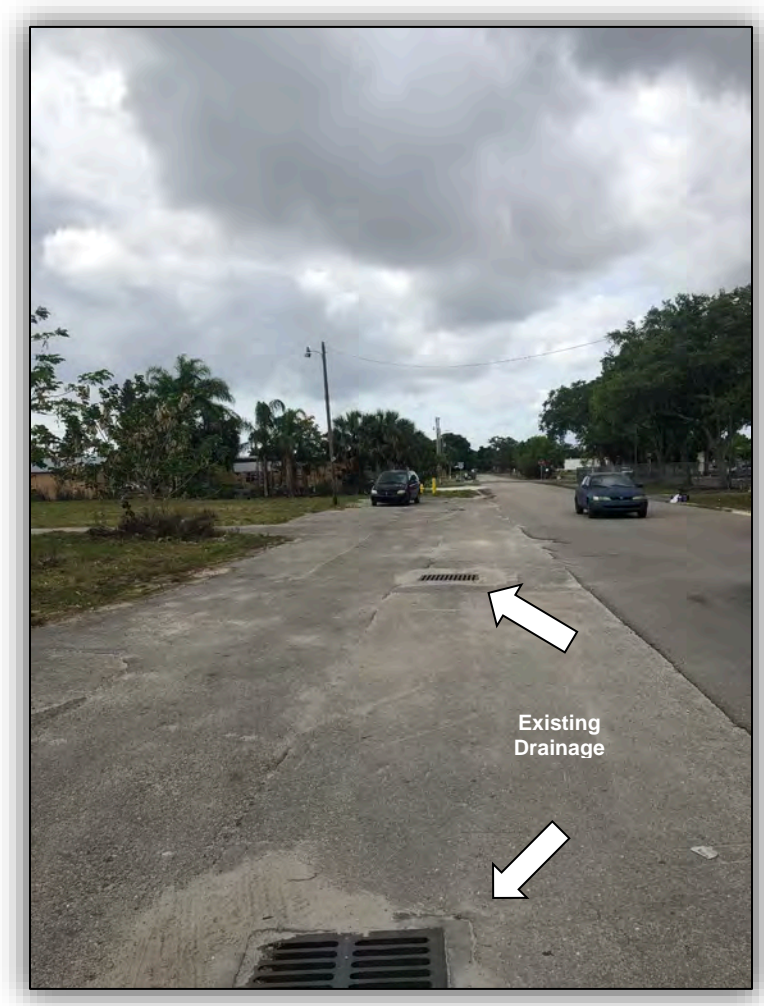
Figure 12-1: Existing Drainage on East Side of South 4 th Street
