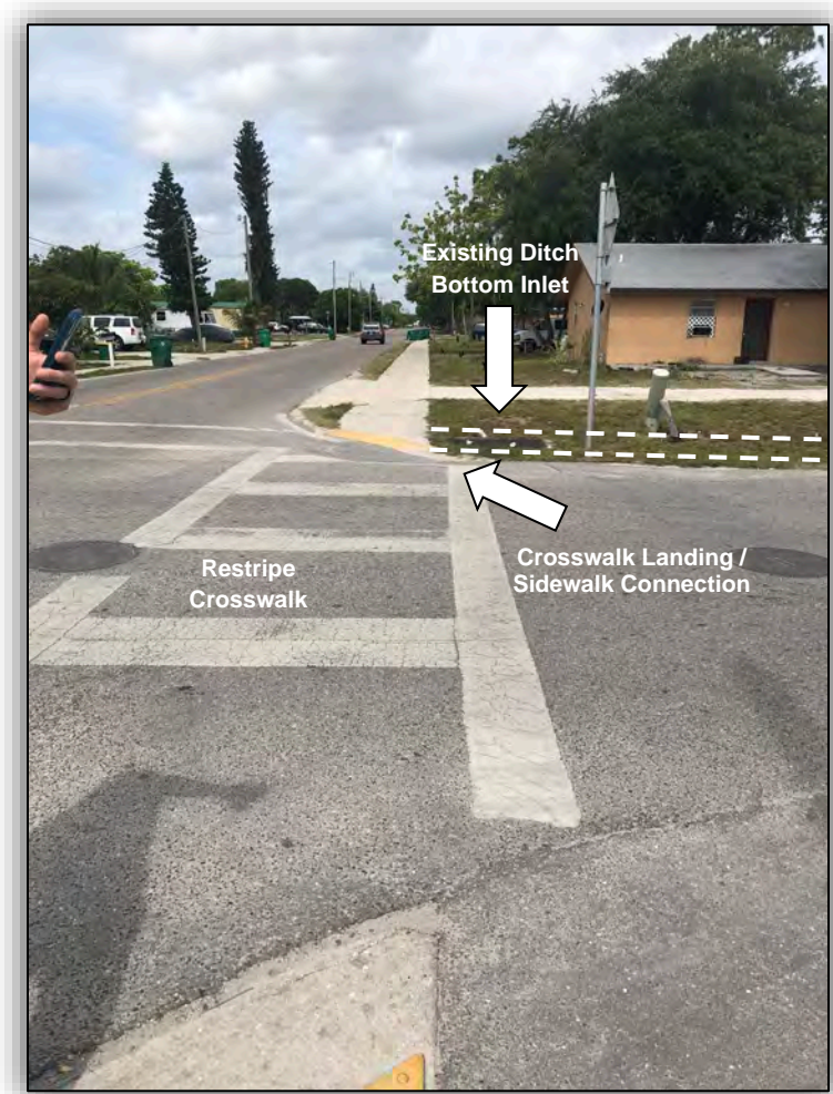
Figure 11-1: Sidewalk Connection / Crosswalk at South 3 rd Street and Colorado Avenue
