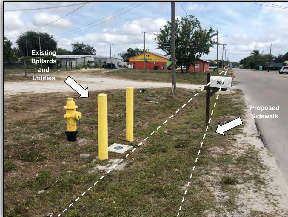
Figure 10-3: South 2 nd Street Utilities
