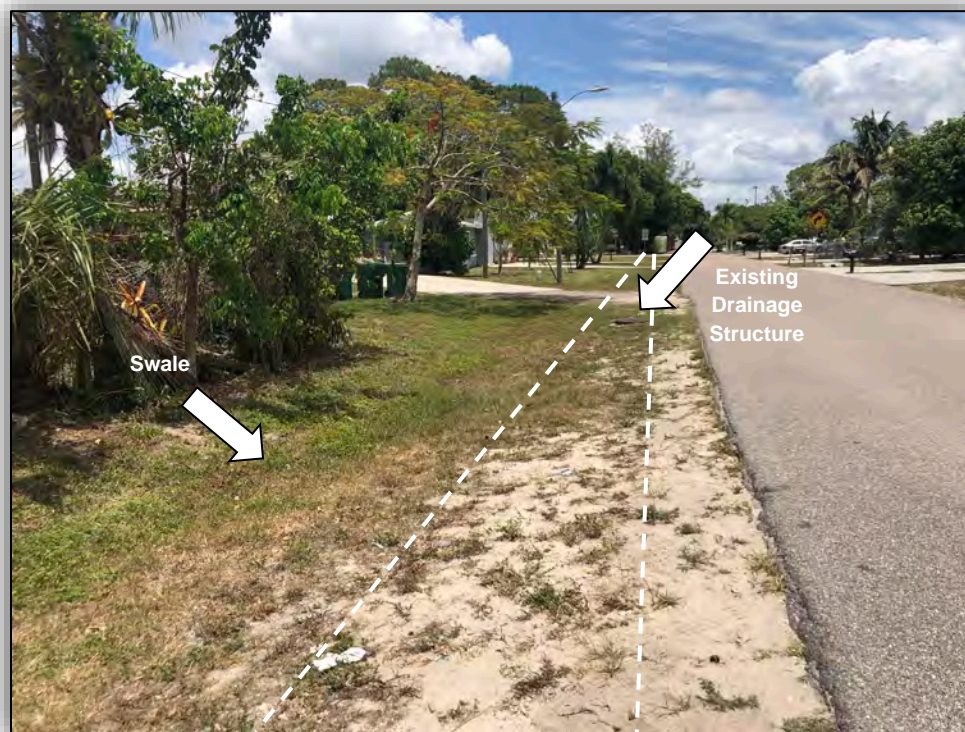
Figure 3-2: McCarty Street North Side
